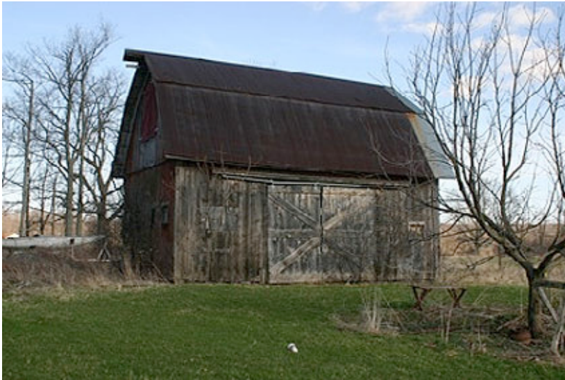
Karen Brummund Storm Road , Groton, NY, before installation
